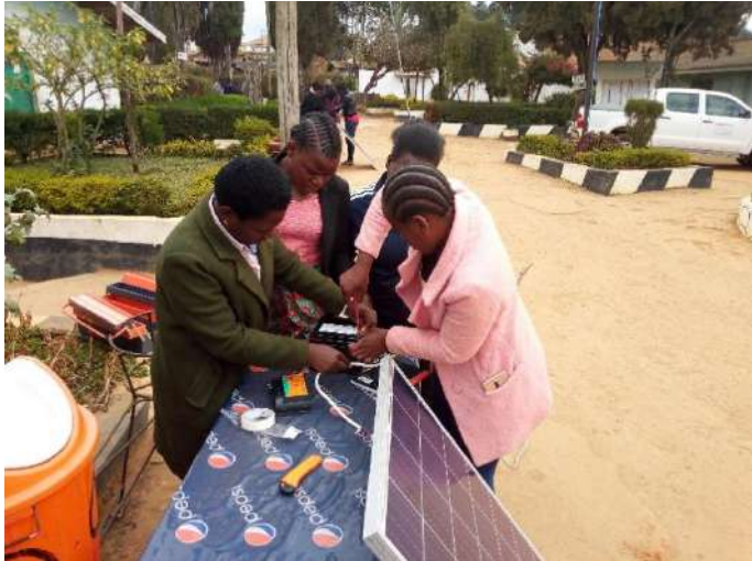
Photo 11: Girls practising solar home system installation in Njombe © TAREA
