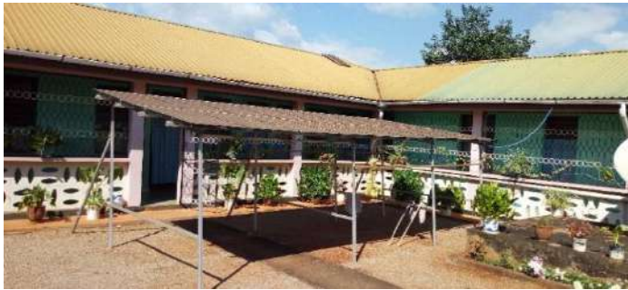
Photo 17: 2.96kWp solar system at St. Ann Sisters, Morogoro ©TAREA
